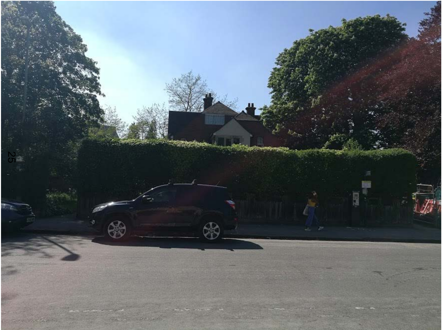
Elevation of Warham House to Mansfield Rd, Copper Beech and Chestnuts retained (RHS)
