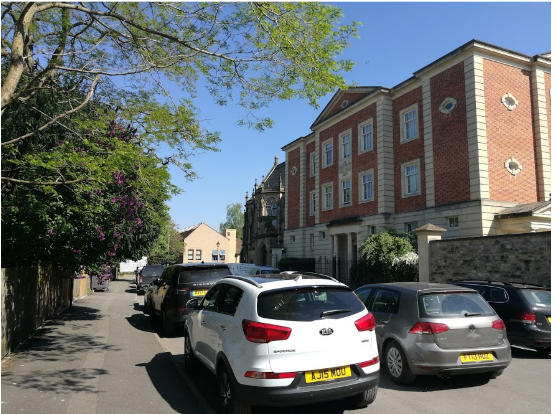
View of buildings opposite Warham House and No.1 Savile Rd
