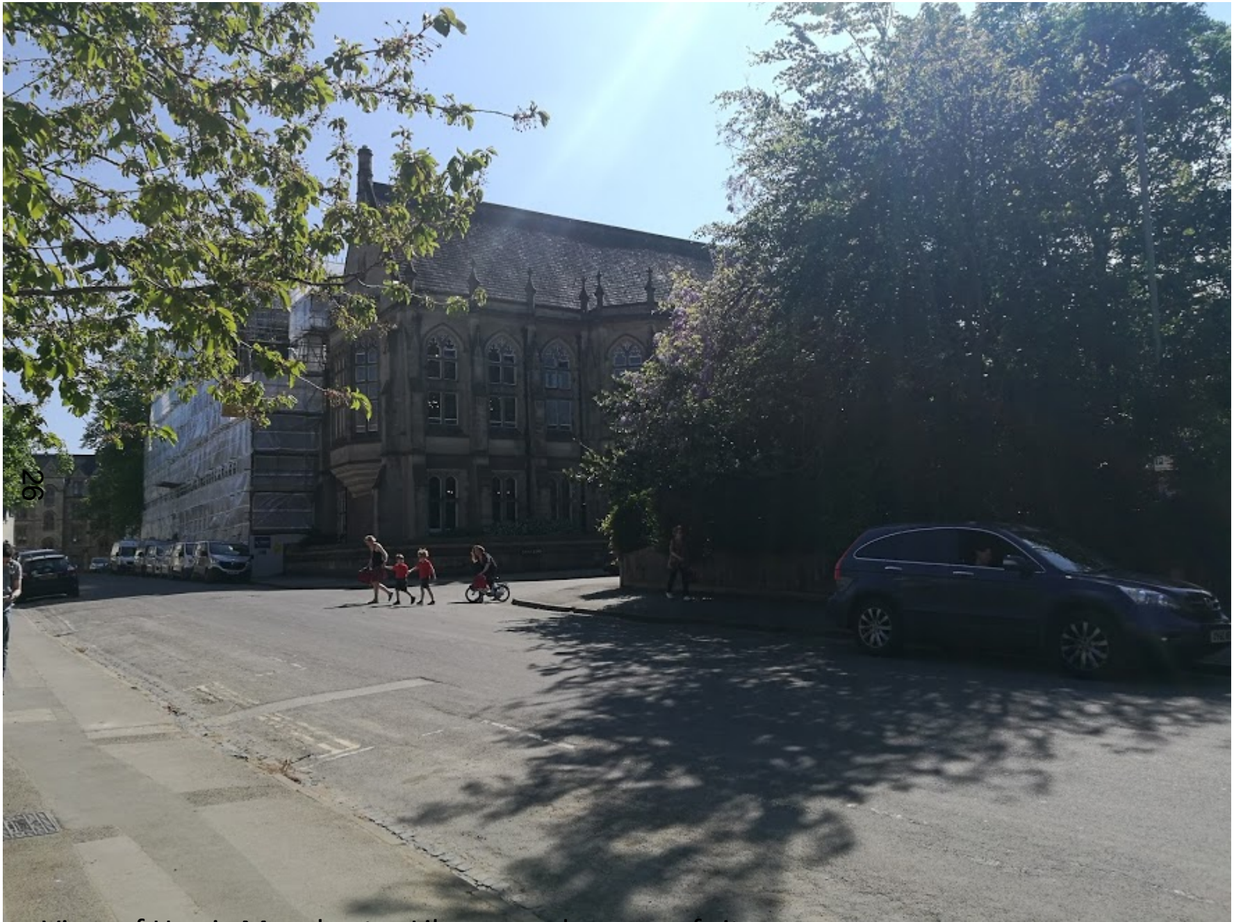
View of Harris Manchester Library and corner of site
